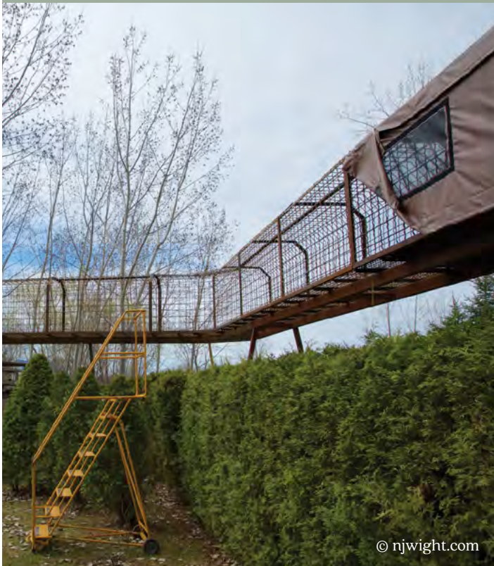
Our skywalk expansion is almost complete!
